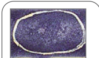
Hose with cover charred area from high heat or extreme aging due to heat or ozone
