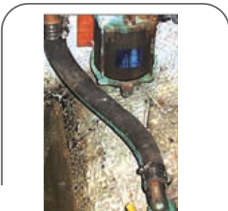
Clamps installed with screw tightening heads in line. It is recommended to offset as see below.
